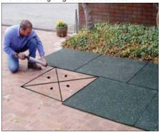
Installation must be to a stable surface. This can be by complete or partial direct gluing to a suitable existing surface or involve the creation of a smoothed and stabilised compacted crusher dust base with minimum 2% crossfall.
